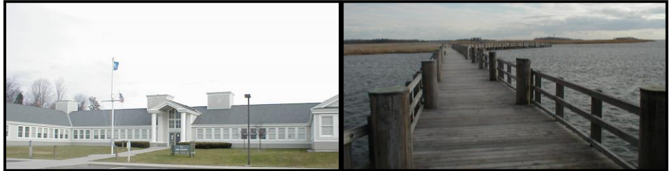
Fishing Pier, Boardwalk and DEEP Marine Fisheries Headquarters and Boating Division, Ferry Road, Old Lyme, CT
