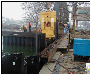
NLDC Bulkhead Replacement, New London, CT
