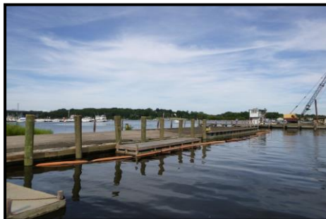
Wharf Stabilization, Old Saybrook Town Dock, CT
