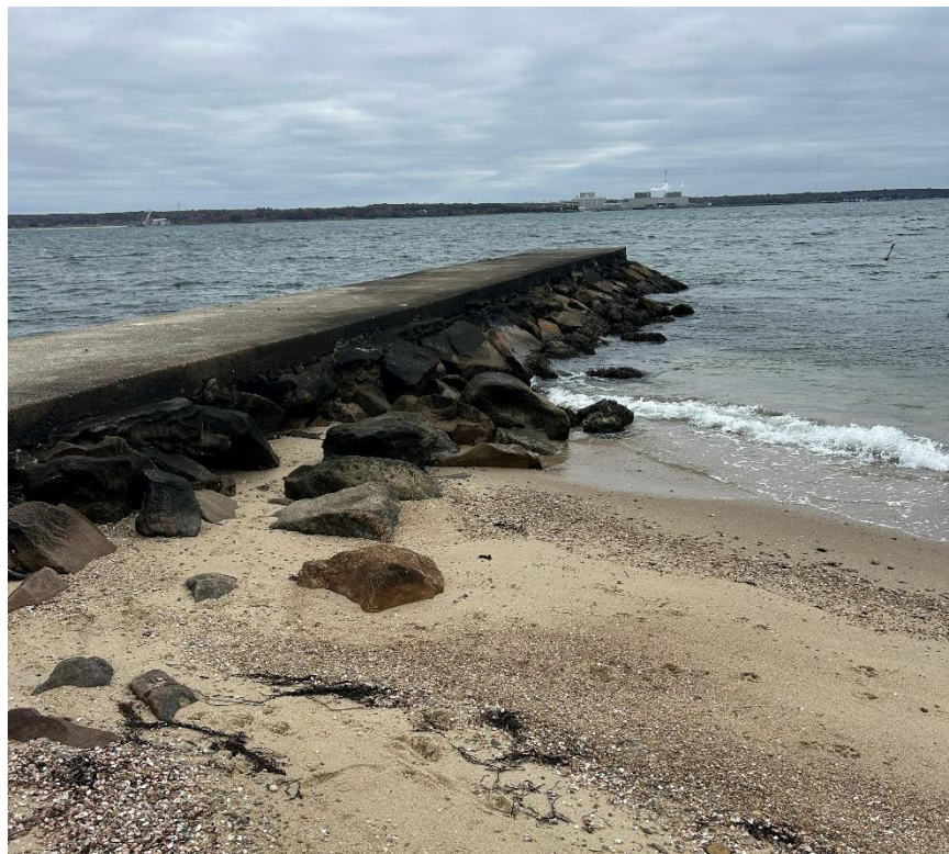
Photo 25: Sea Breeze pier South side armor stone
