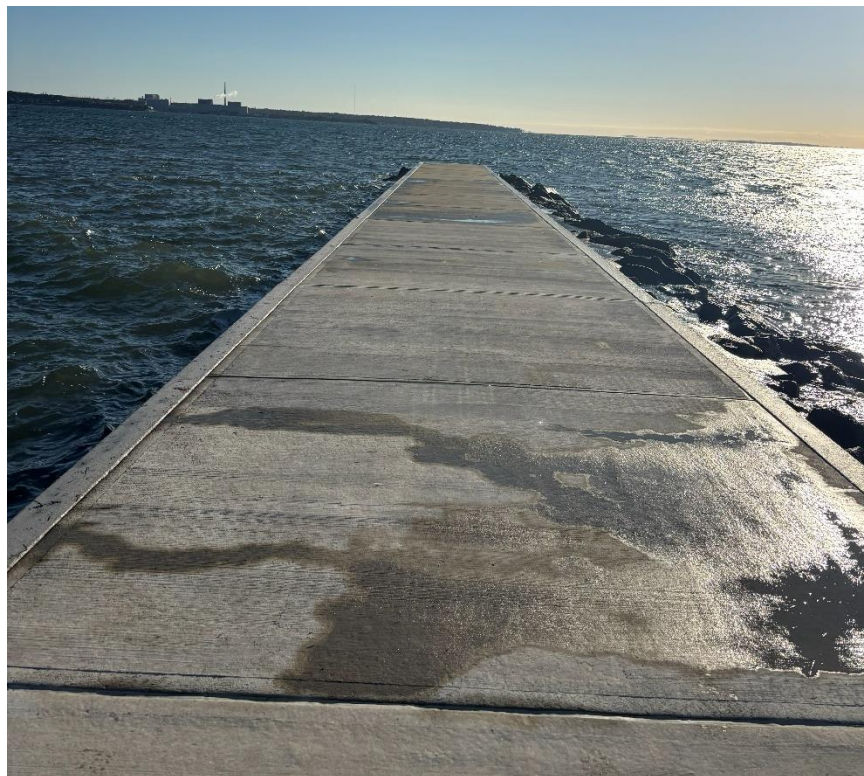
Photo 15: Indianola steel pier concrete walkway
