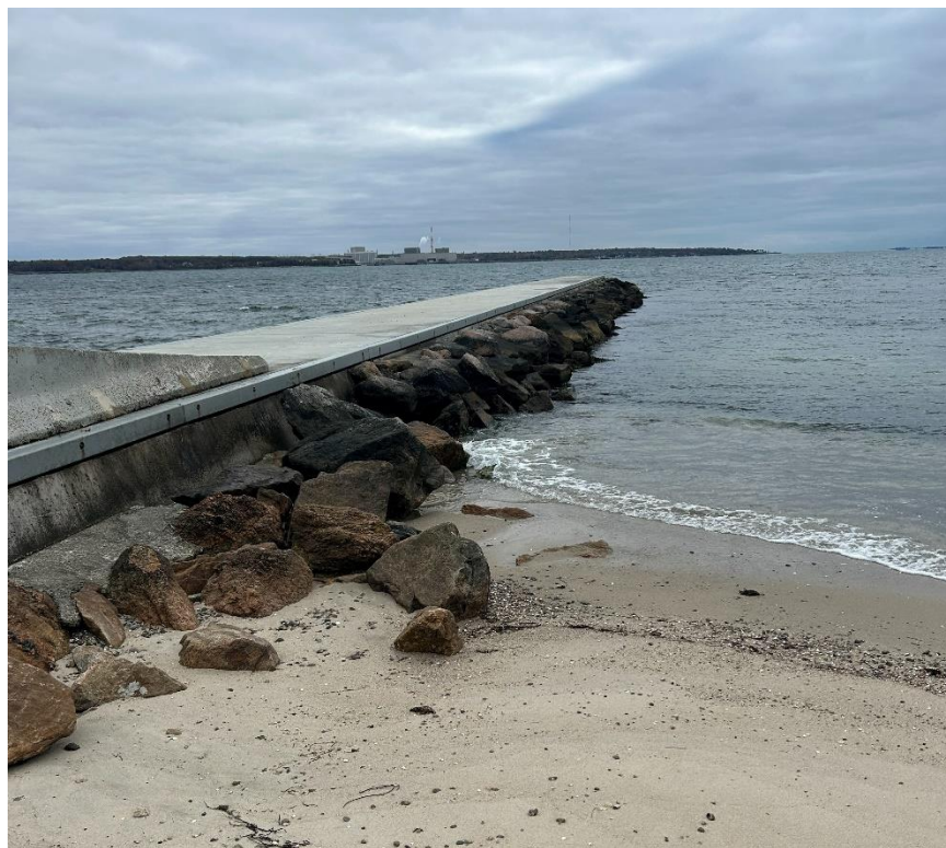
Photo 12: Indianola steel pier South side
