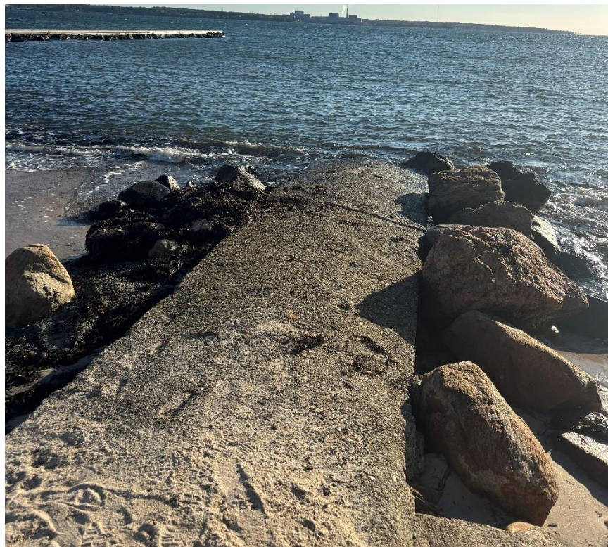
Photo 18: White Cap access way drainage pipe encasement
