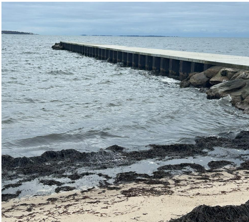
Photo 10: Indianola steel pier North side
