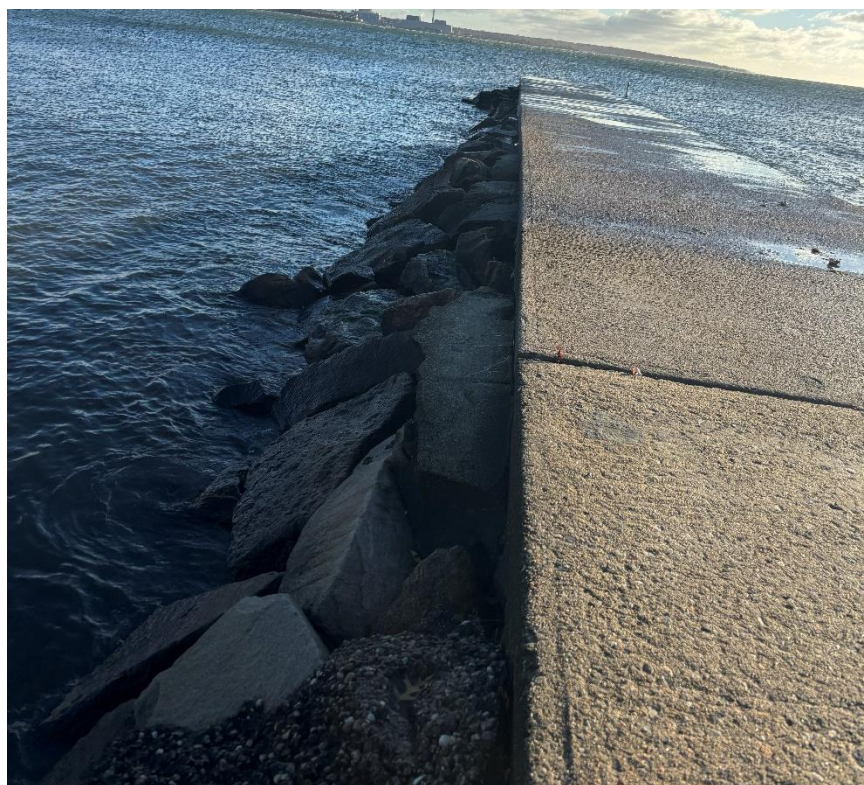
Photo 26: Sea Breeze pier North side armor stone settlement
