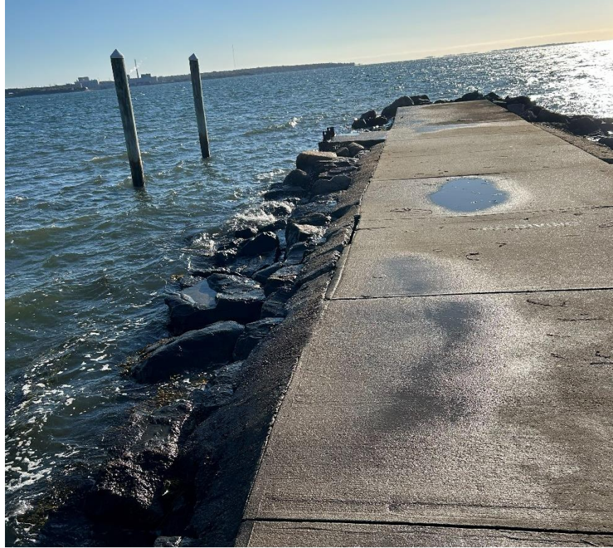
Photo 3: Nehantic pier North side end
