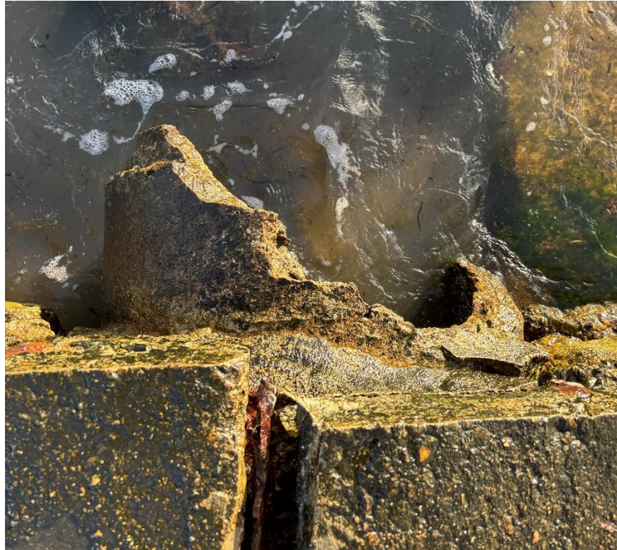
Photo 19: White Cap access way drainage pipe end
