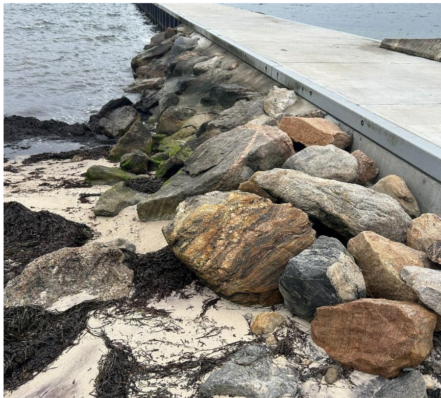
Photo 11: Indianola steel pier North side armor stone
