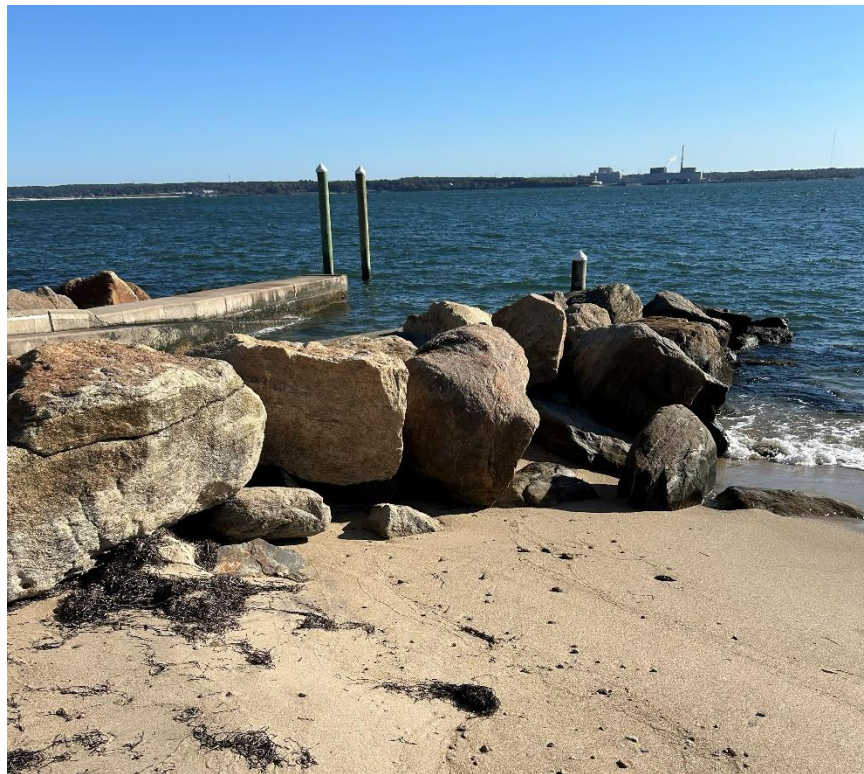
Photo 32: Sea View boat launch South armor stone
