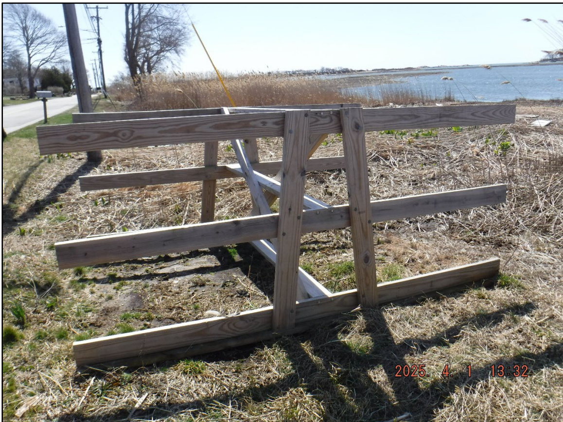
View of existing kayak rack from upland, looking south.
