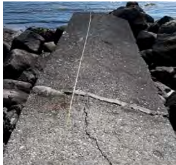
Drainage Pipe Concrete Encasement
