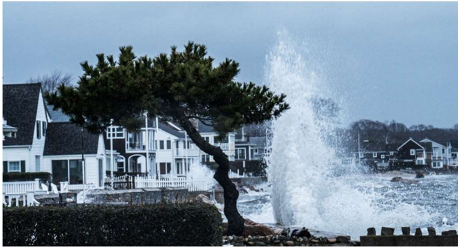
Image 21: Waterfront looking north; approximately Sea Spray ROW (December 2022)
