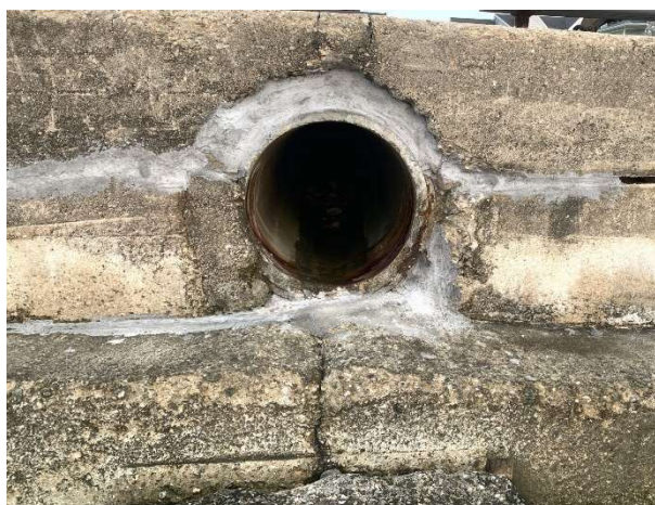
Image 19: Drain outfall (Blue Heron Way, 2023)
