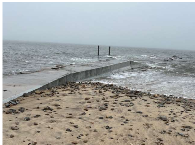
Image 7: South Beach groin, January 2024 (image courtesy of Jan Orsini)
