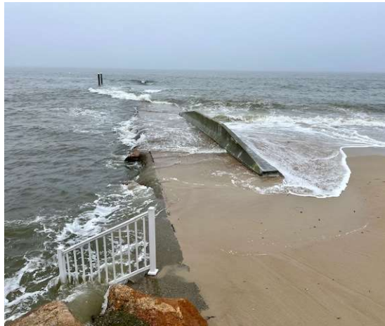
Image 6: Nehantic groin, January 2024 (image courtesy of Jan Orsini)
