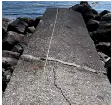
Drainage Pipe Concrete Encasement
