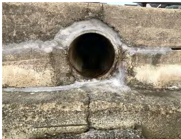
Image 15: Drain outfall (Blue Heron Way, 2023)
