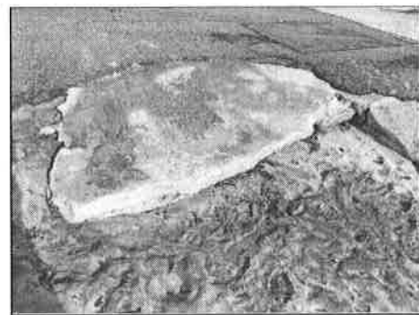
At Sea View Boat beach. Cut, remove slab and replace with sloped concrete.
