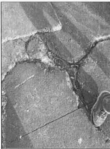
This is a Sea Breeze/Sea View walkway. Form, fill concrete and level/square off.
