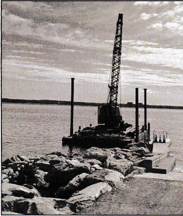
5/19/21 - New piling installed.
