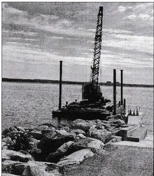
5/24/21 -Installed piling at Sea View.
