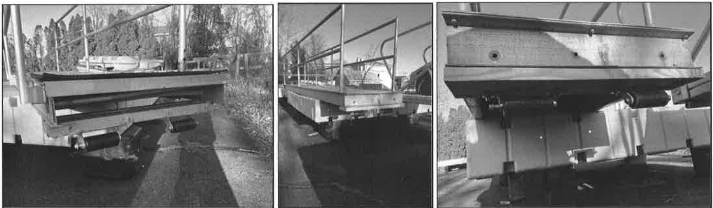
The Crew (Will, Mike, Skip, Jim Allen) installed new rollers on the gangways - saving hundreds of $$.
